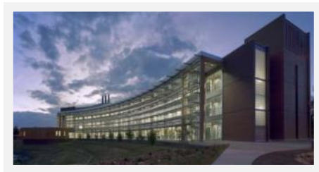
上图北亚利桑那大学综合实验楼 (Applied Research and Development)
