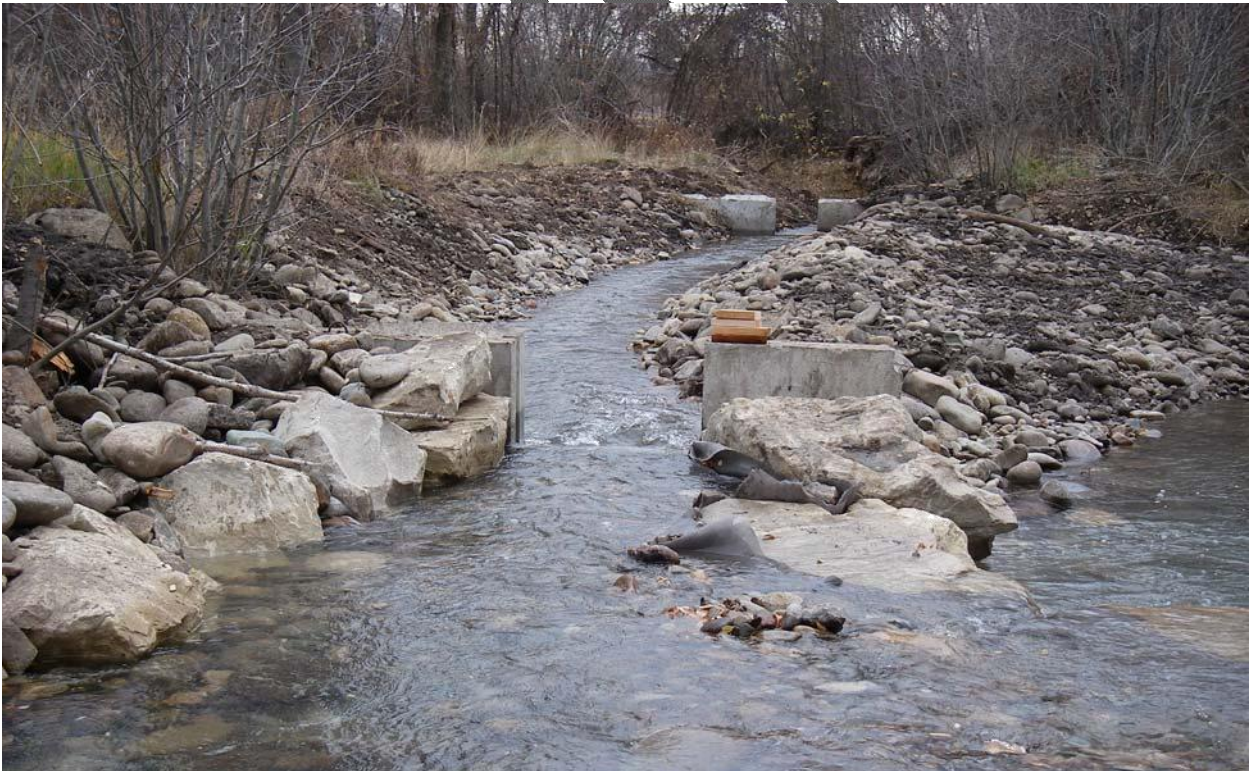
POST: Downstream view of ditch inlet (left) and river channel (right).
