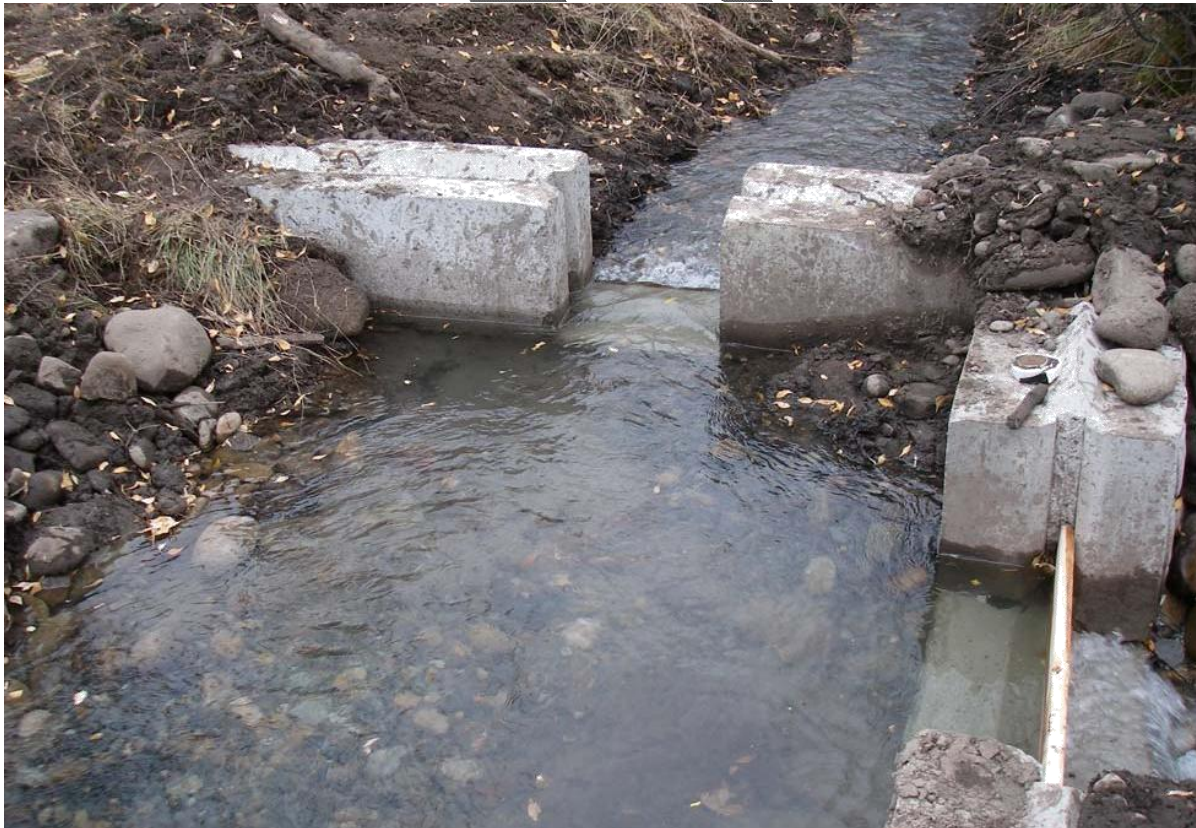
POST: Downstream view of new heading (left) and sluice opening (right).
