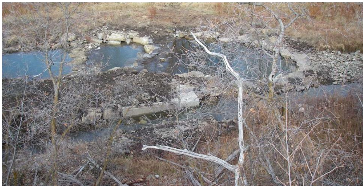
POST: Hillside view of diversion inlet and cross vane structures (river flow is right to left).
