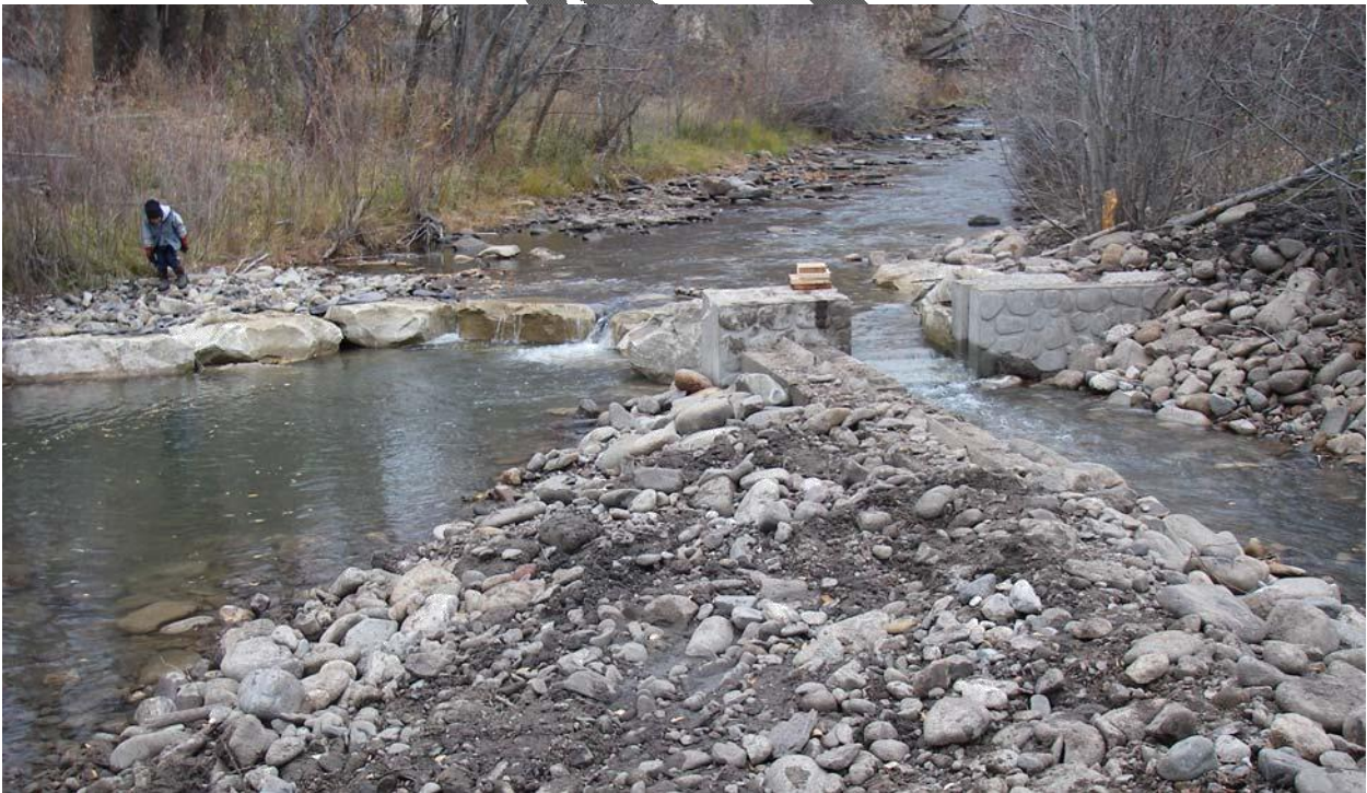
POST: Upstream view of diversion inlet, diversion channel and cross vane structure.
