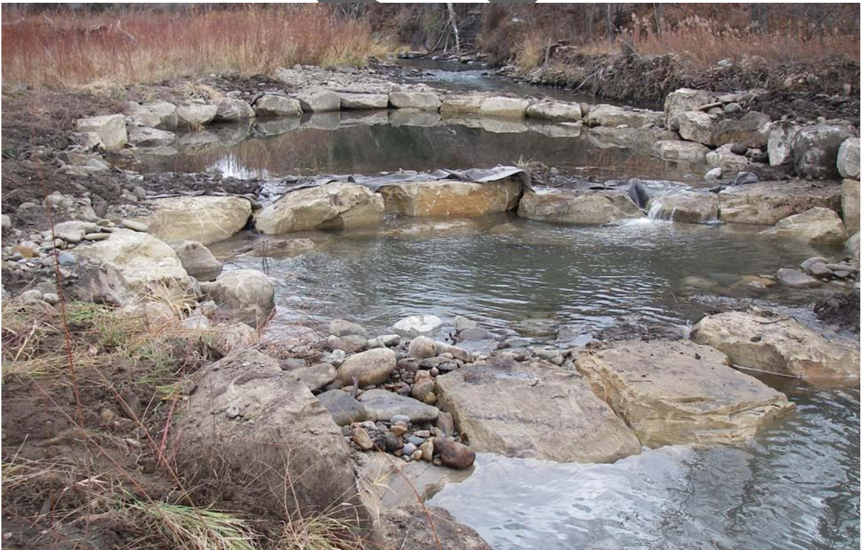
POST: Upstream view of cross vane structures.
