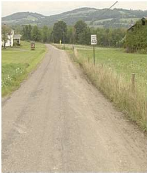
An illustration: SR 3020 in Towanda Township, Bradford County, Pennsylvania after a high volume of overweight drilling trucks and a Northeast winter (Photo: PennDOT Engineering District 4-0)
