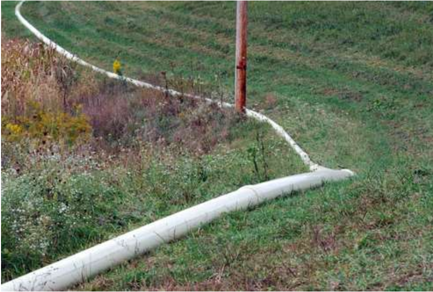
Figure 2: Temporary Piping Carrying Flow back Water to a Holding Pit in Pennsylvania – (Source: Marcellus-Shale 2013).
