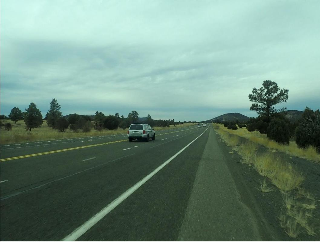
Wide shoulder along Route 64 where the speed limit is 65 mph and the road switches between 2, 3, and 4 lanes. The shoulder is this wide for roughly 70% of the distance between Spring Valley Road (forest road 141) and Interstate 40.
