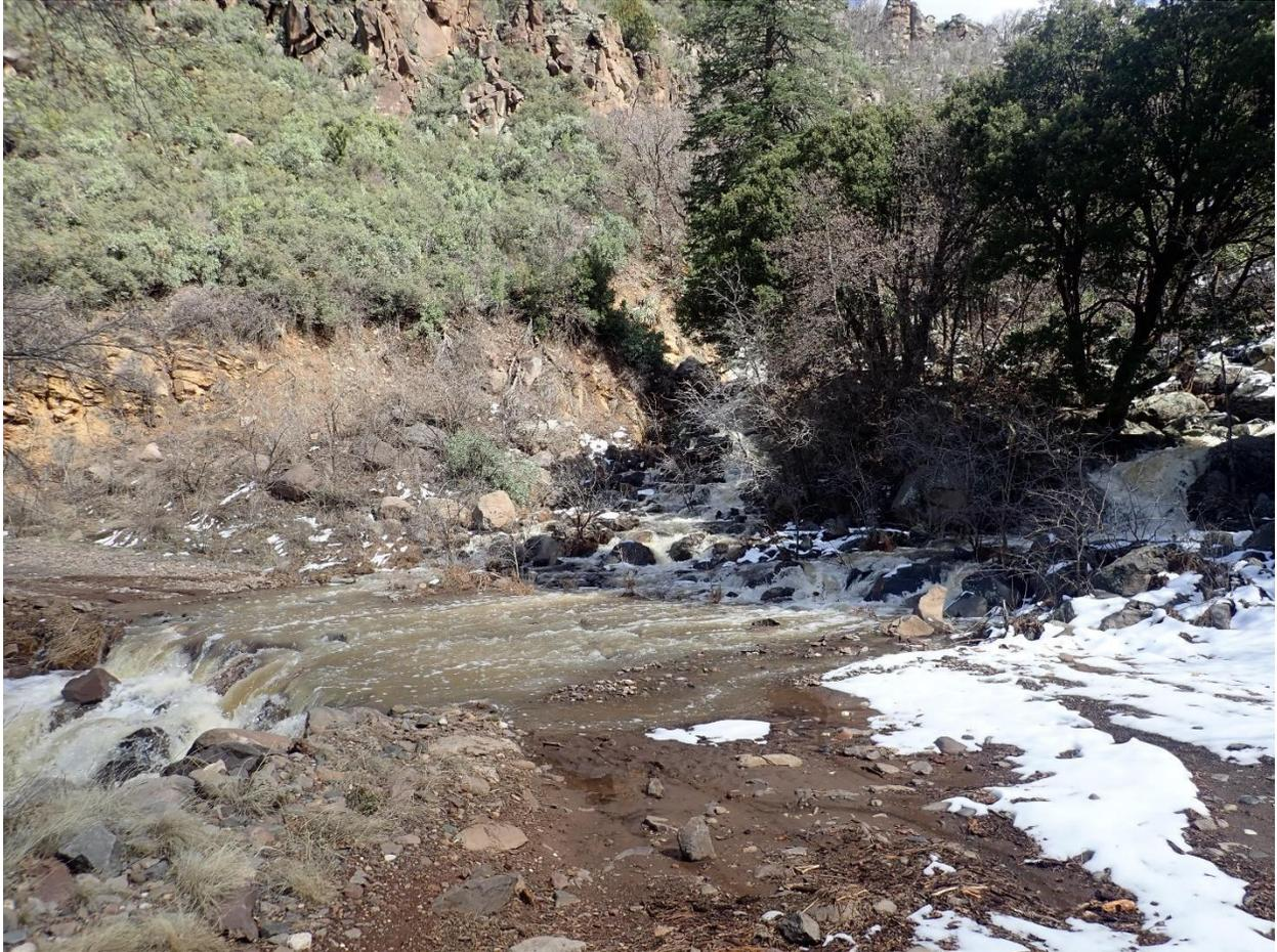
This picture shows Casner Canyon 1 on Schnebly Hill road taken on 3/21/2020. The water was flowing quickly and eroding the road. The water is crossing the road perpendicularly on a hairpin corner and is roughly 20-30 feet wide and up to 36" deep in places. The water depth looks minimal in the photo. The field researcher found this depth out the hard way when he attempted to cross the flow by bike.
