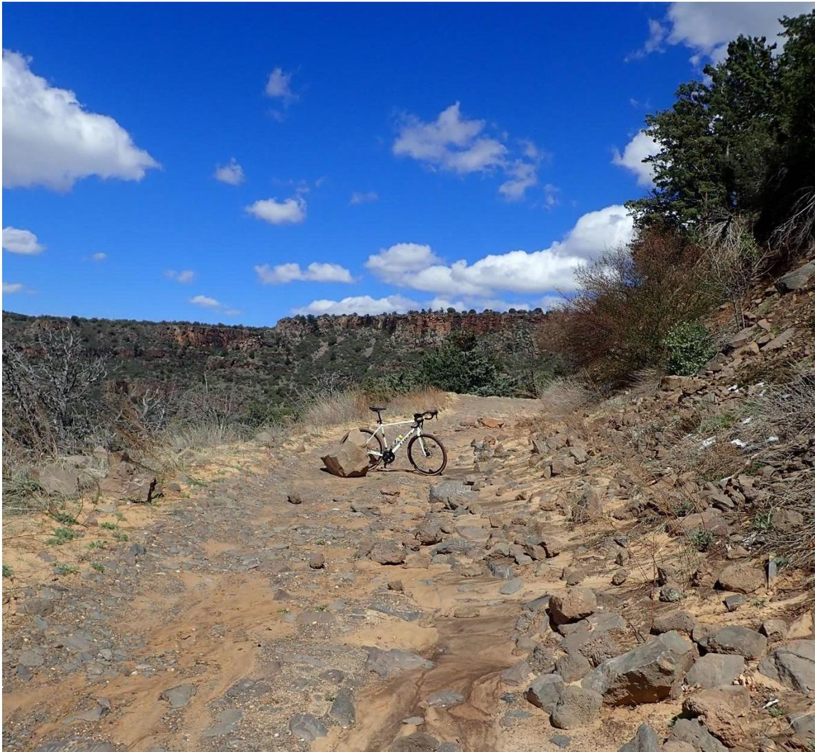
This image shows one of a few rockslides on Schnebly Hill road above the seasonal vehicle closure. The rock debris is seen on the right side of the road and the field researcher's bicycle is leaning against a large boulder that was likely part of the rockslide to provide scale.
