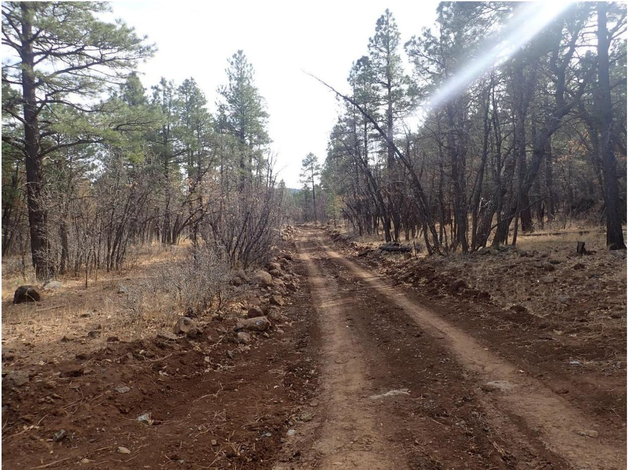
This photograph was taken by the field researcher looking south on Forest Road 132D. It shows a section of road that appeared to be hastily graded possibly during wildfire mitigation. Though it may not appear significant the rocks dislodged by the grading made this section painstakingly slower than the rest of the route.
