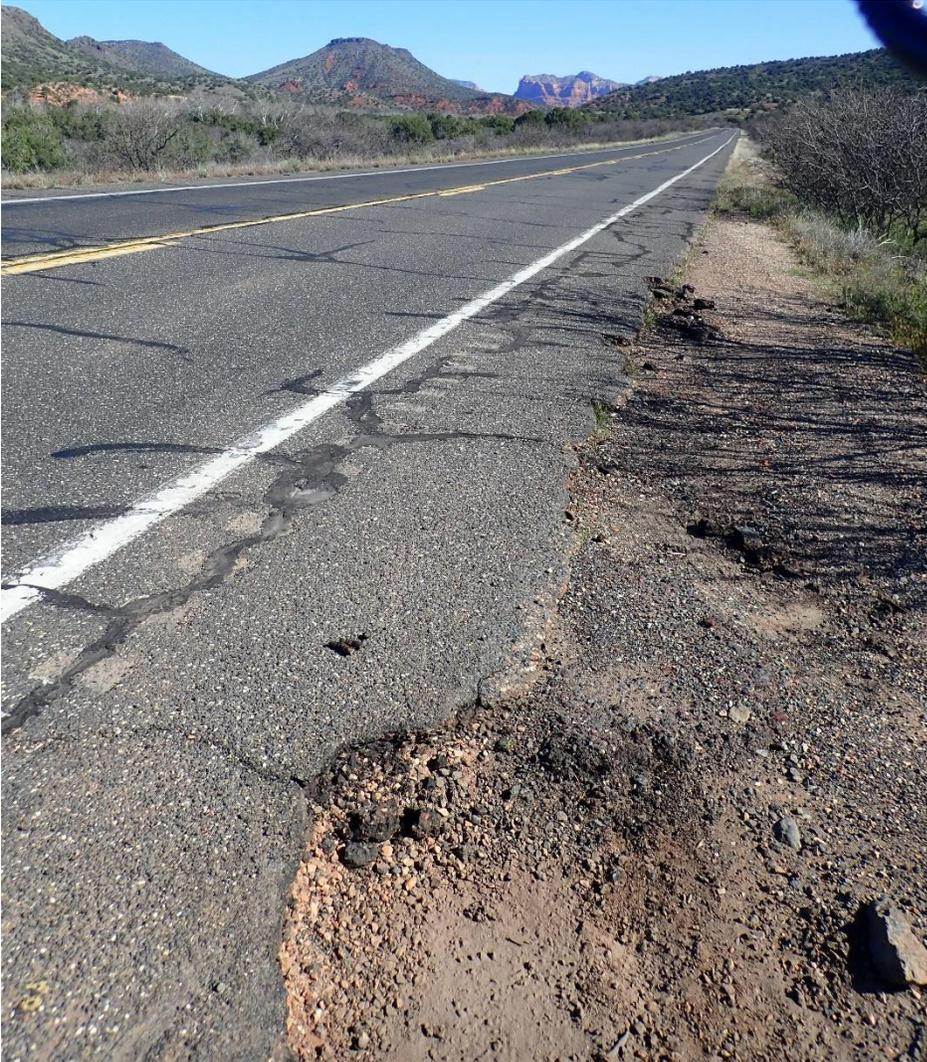
This image shows a section of narrow, eroded road shoulder along highway 179. The picture was taken looking northbound roughly 3 miles south of the Village of Oak Creek. Directly to the right of the white line in the foreground a rumble strip limiting the width of the shoulder for bike tires can be seen.
