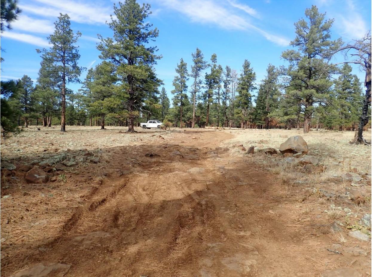
This photo illustrates the transition to the less maintained portion of Forest Road 132D once inside the Pinegrove Quiet Area. Particularly note the significant ruts and medium size rocks on the road surface.
