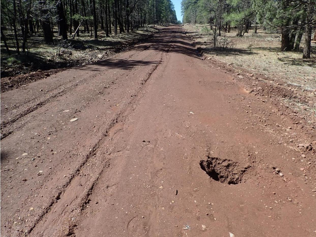
This picture shows a hole in the road where a metal corrugated culvert pipe for drainage caved in. The pipe runs perpendicularly under the road and appeared to collapse due to vehicles traveling on the road with the wet soft conditions.
