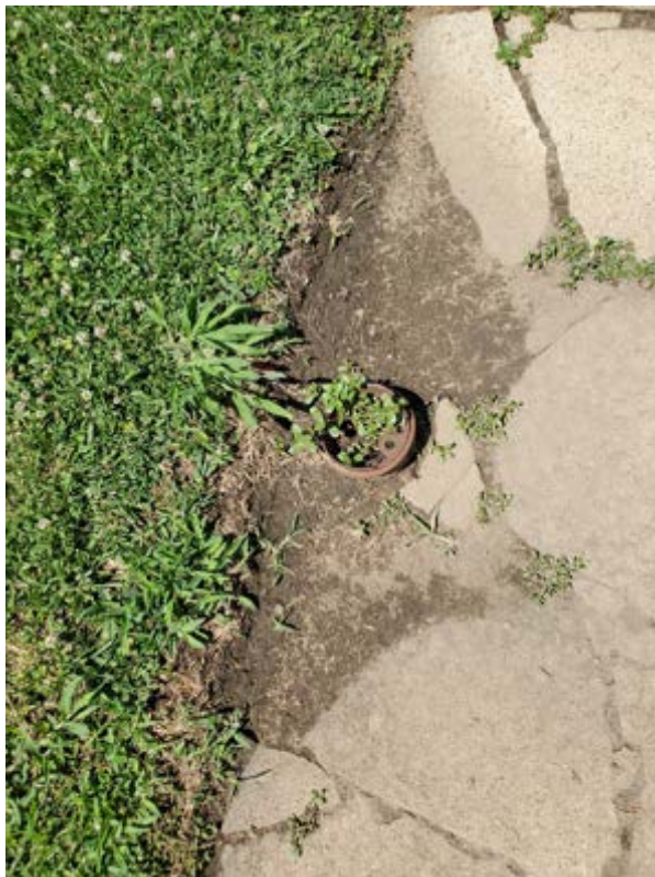
Figure 31 Exposed water valve in sidewalk. Source: CAR Participant, 2019
