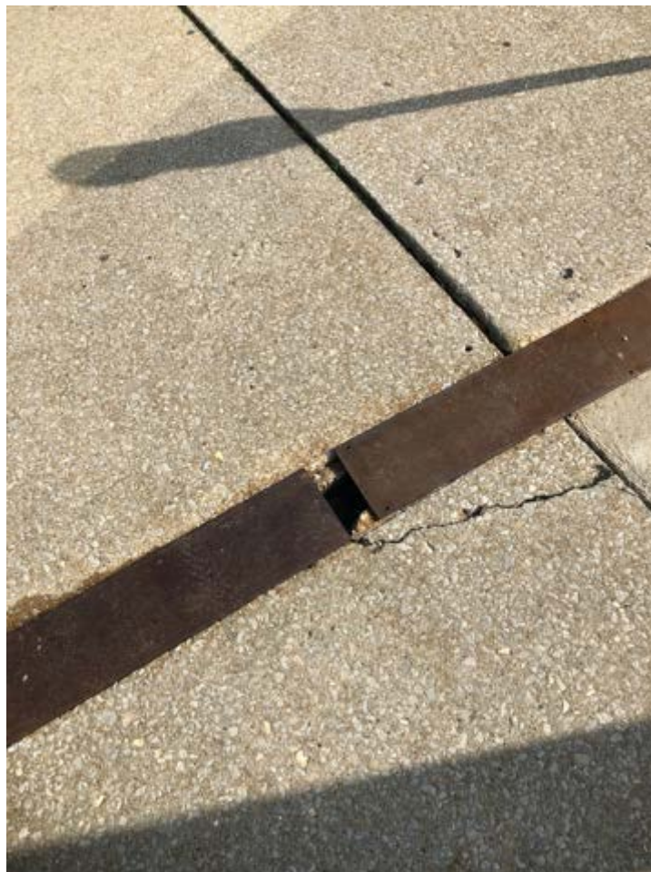
Figure 35 Exposed drainage pipe cover in sidewalk. Source: CAR Participant, 2019
