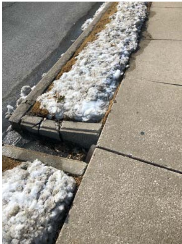
Figure 37 Exposed drainage pipe with 4-inch drop to asphalt. Source: CAR Participant, 2019
