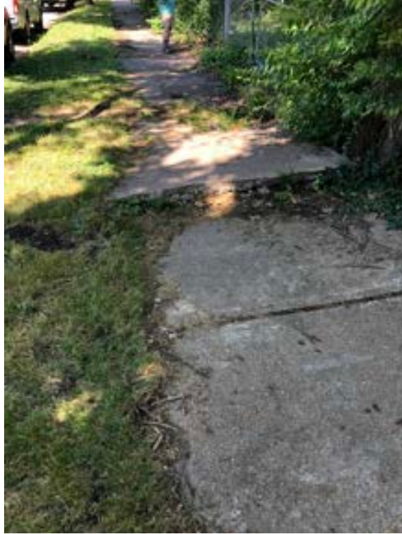
Figure 28 Cracked and heaved Sidewalk ~1.5 inches above grade. Source: CAR Participant, 2019
