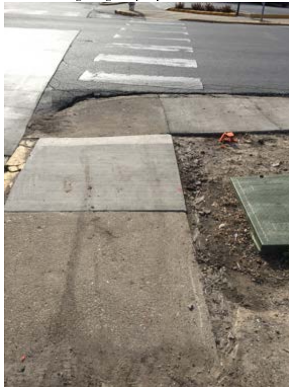
Figure 57 Trip hazard transition to road and transition from sidewalk to asphalt not level. Source: CAR Participant, 2019
