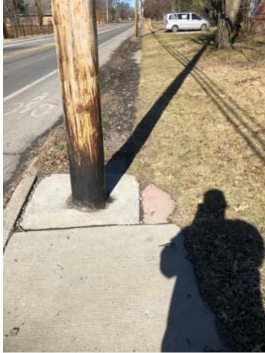
Figure 41 Phone poll in middle of sidewalk, sidewalk less than 4 feet wide, and mud-covered sidewalks. Source: CAR Participant, 2019
