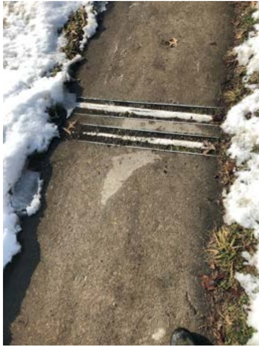
Figure 38 Exposed drainage pipe in sidewalk. Source: CAR Participant, 2019
