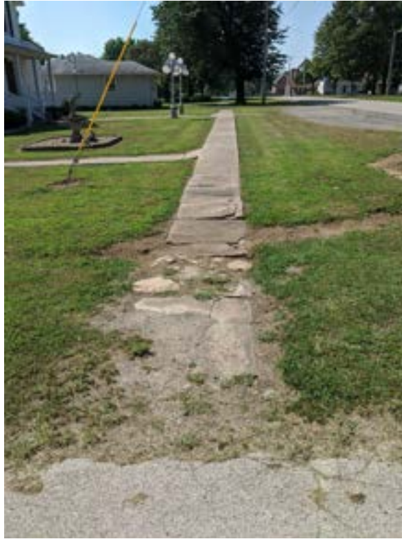
Figure 30 Cracked and degraded sidewalk. Source: CAR Participant, 2019
