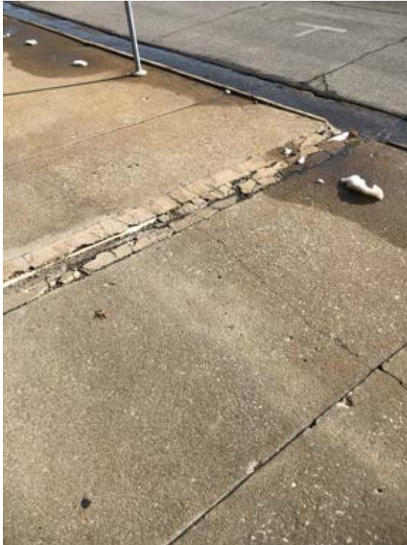
Figure 36 Exposed drainage pipe and cracked area around pipe. Source: CAR Participant, 2019
