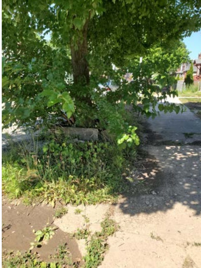
Figure 40 Vegetation obstructing sidewalk path and cracked sidewalk. Source: CAR Participant, 2019.
