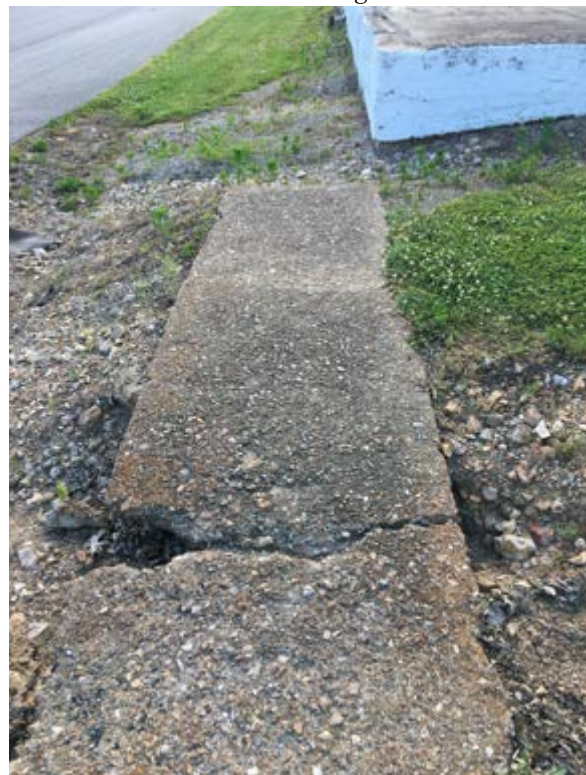
Figure 29 Cracked sidewalk with no connection. Source: CAR Participant, 2019
