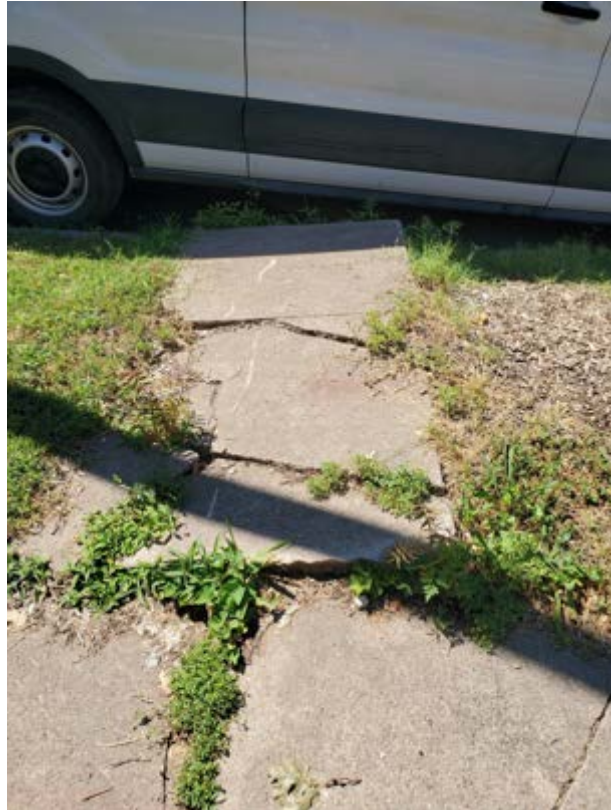
Figure 27 Cracked and heaved sidewalk.
