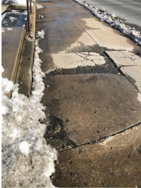
Figure 26 Cracked Sidewalk and snow coverage. Source: CAR Participant, 2019
