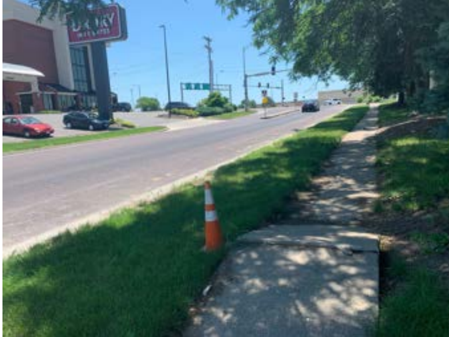
Figure 21 Heaved Sidewalk ~3 inches above grade. Source: CAR Participant, 2019
