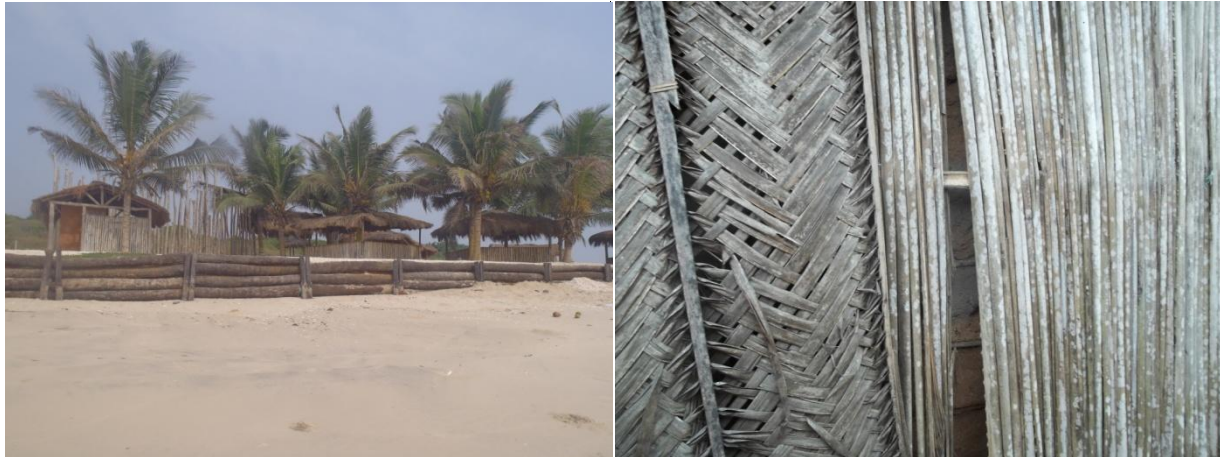
Figure 10: Coconut retaining wall, and live palms used for shade. The structures used coconut stems as the posts and the rachis from the frond, and the fronds woven together, to construct the walls. Location: outside of Gomwa Nyanyano, Central region, Ghana, West Africa. (photo taken by Ben Ross Caulum)
