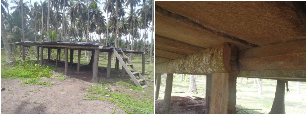
Figure 11: Coconut stems used as pillars and cut into timbers for the construction of a raised patio. Location: Outside of Atuabo, Western region, Ghana, West Africa (photo taken by Ben Ross Caulum)
