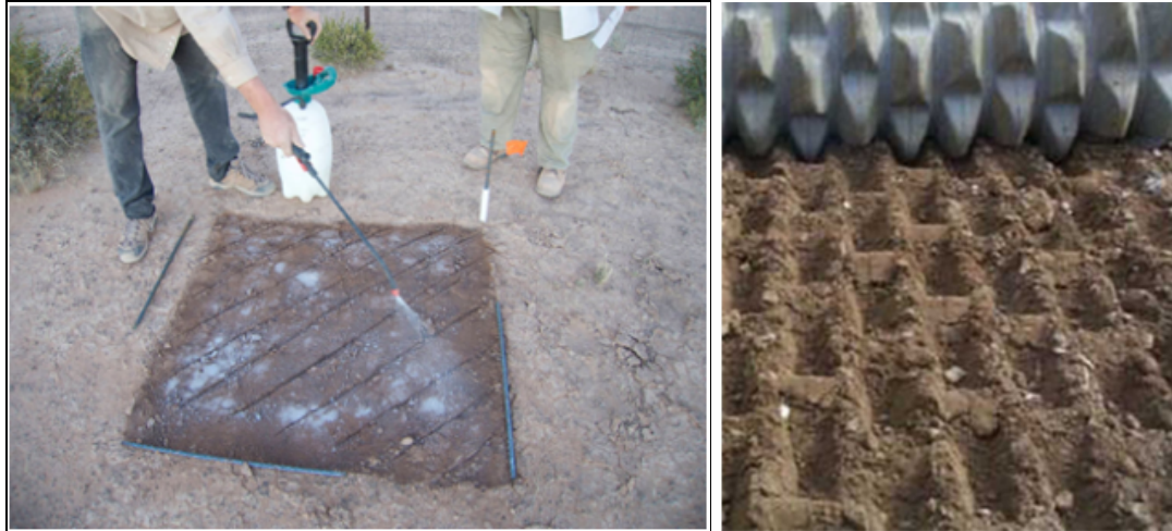
Figure 9. Surface roughening and polymer application (left, credit A. Antoninka) and soil imprinting (right).
