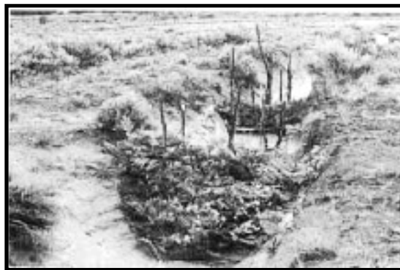
Figure 2.6b: Brush weir example by Zuni farmers. (Norton, Bowannie, Peynetsa, Quandelacey & Siebert, 2002).
